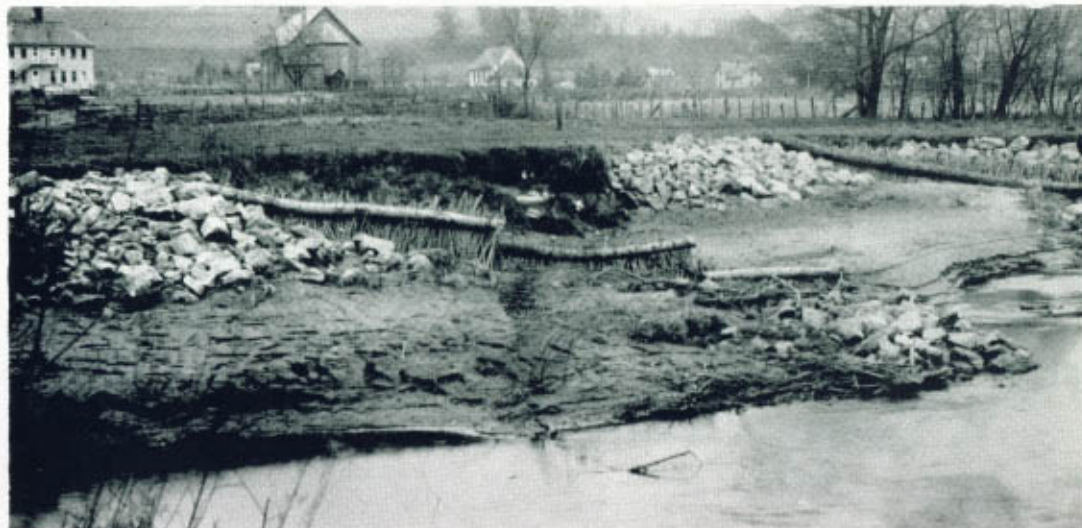
(Above) Rock and brush dams to collect silt and control high waters resulting from careless practices on the land above.
